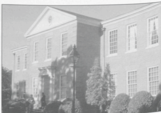
Appleby Hall serves as a classroom building for SEBTC.
