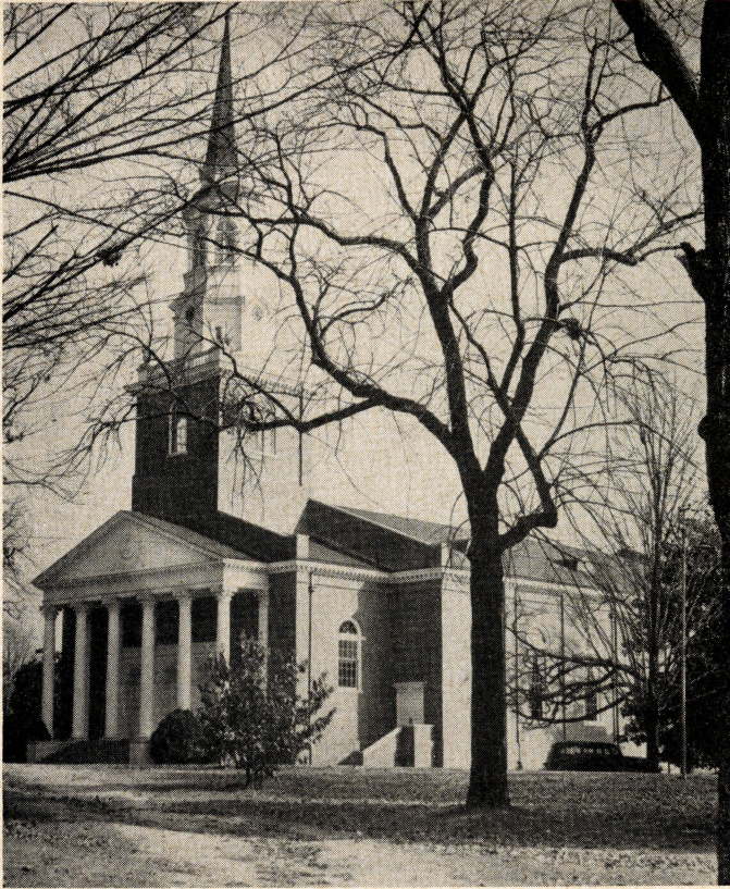
CHAPEL —Due to the primary importance of the Chapel as a worship center of the campus a careful study is being undertaken by a joint committee of the faculty and trustees before plans are made for finishing the interior. At present the Chapel has a temporary ceiling. It is equipped with straight chairs and has only a stage across the front.
