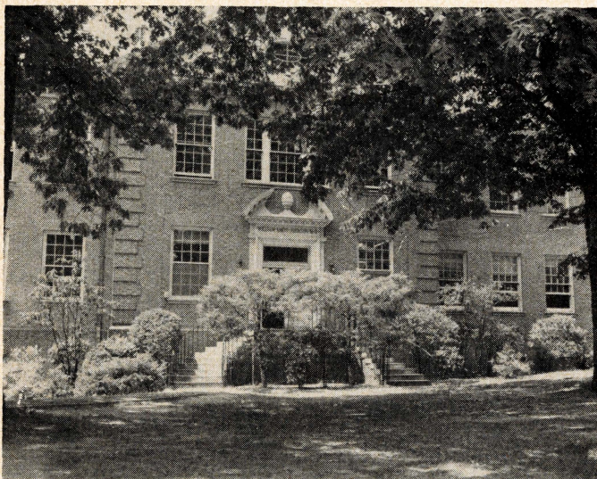
AMOS JOHNSON BUILDING —This building was originally constructed to house the Wake Forest Medical School. The Seminary will make use of it as a classroom building.
