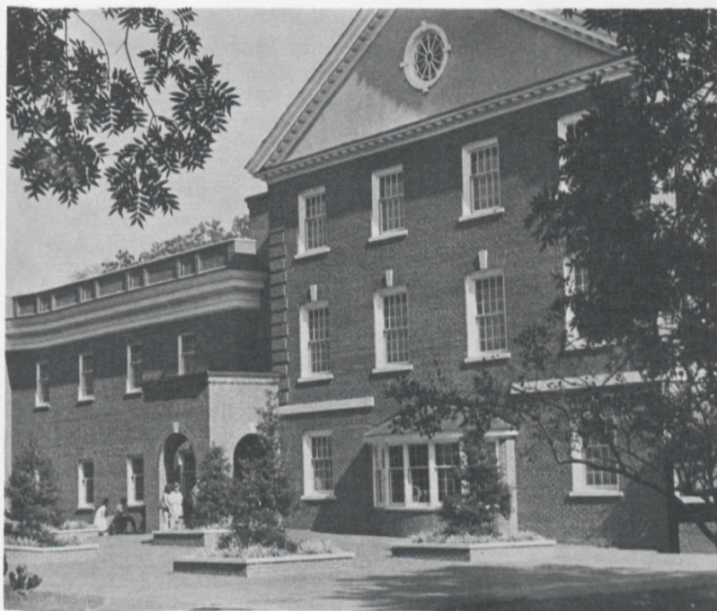
Denny Library Building
